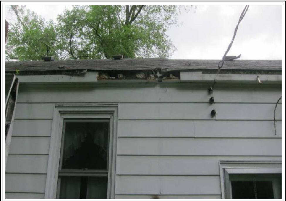
Rear roofline where electrical mast broke off eave and side of dwelling.
