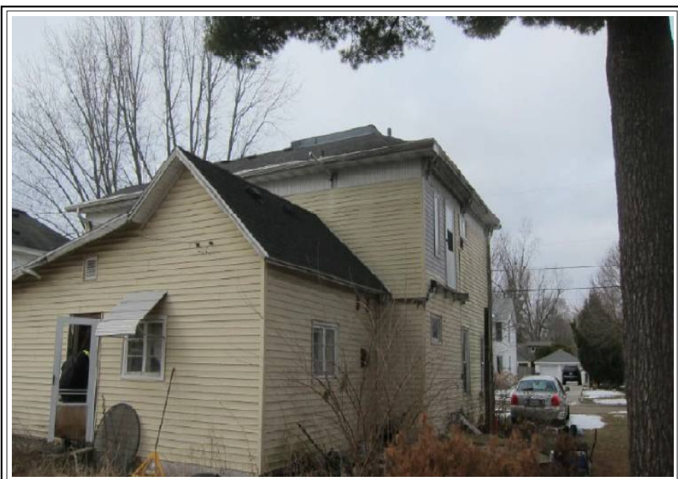
Rear of house
